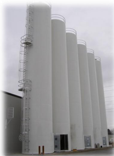
6 Large Silos on Load Stands, Verify Delivery and Usage by Weight
