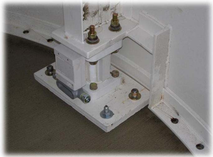
Silo Weight with KM Load Stand is Solid Bolted for Safety
