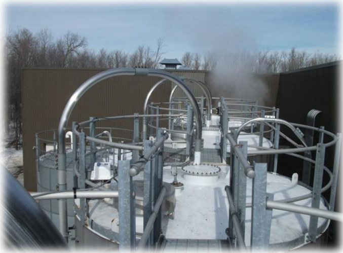
7 Silos with Digital Bindicator GP4 YOYO Inventory System, Networked to all Work Stations in Plant
