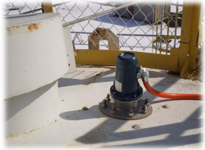
Silo Inventory with No Moving Parts Laser Technology
